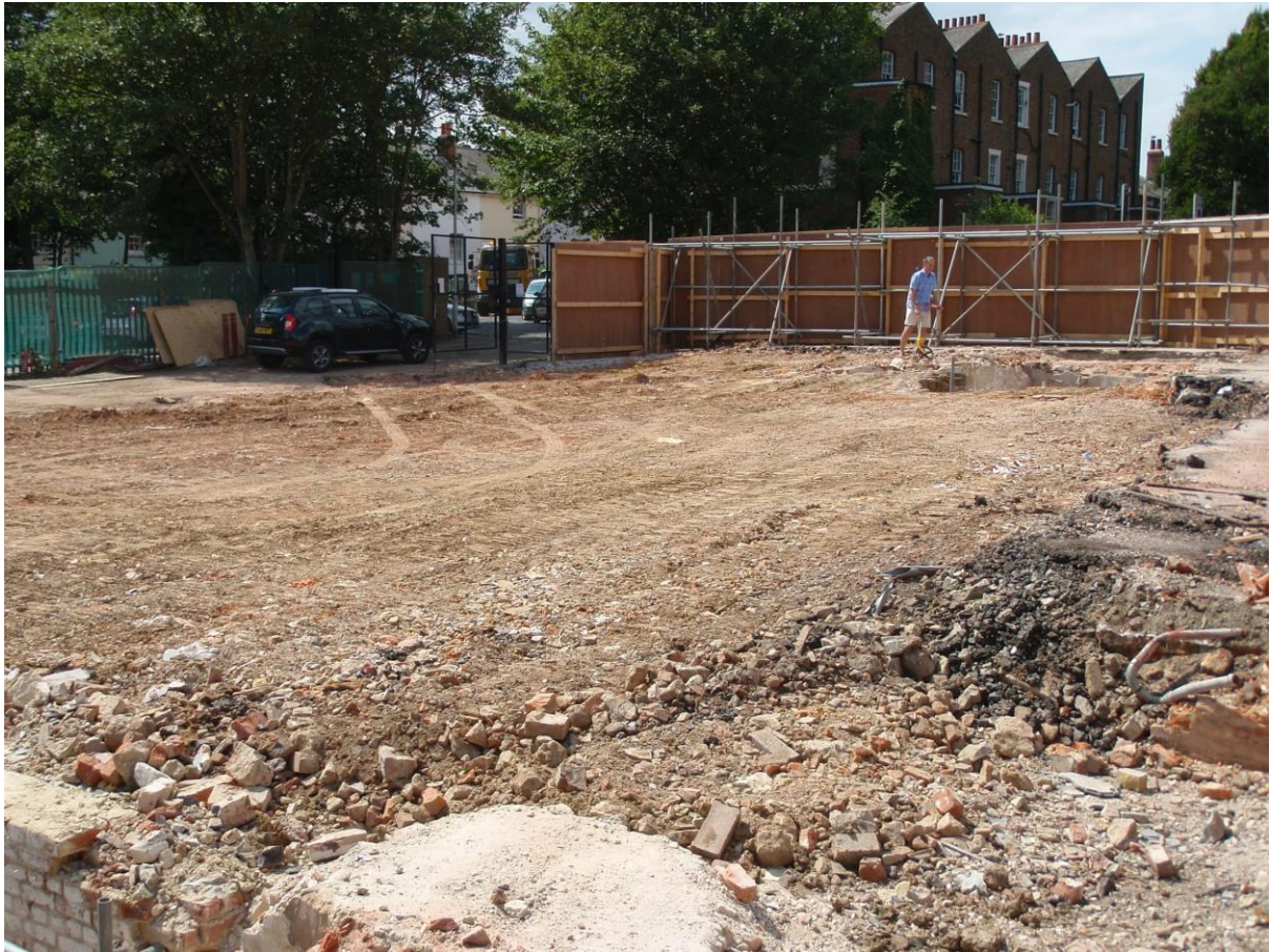
Plate 20. View of demolished site
