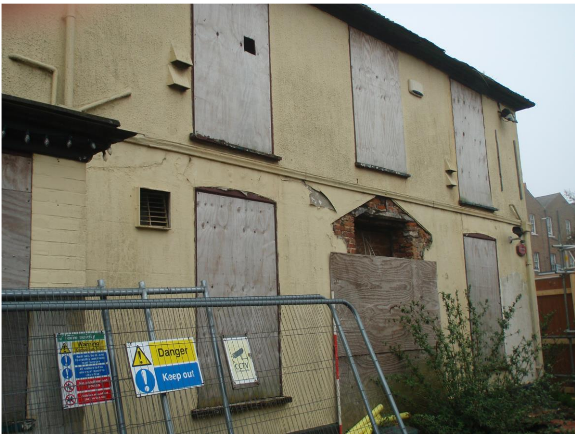
Plate 3. . View of external façade Prince Albert (looking SW)
