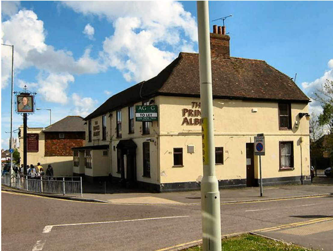
Plate 12. View of façade (c. 1985)
