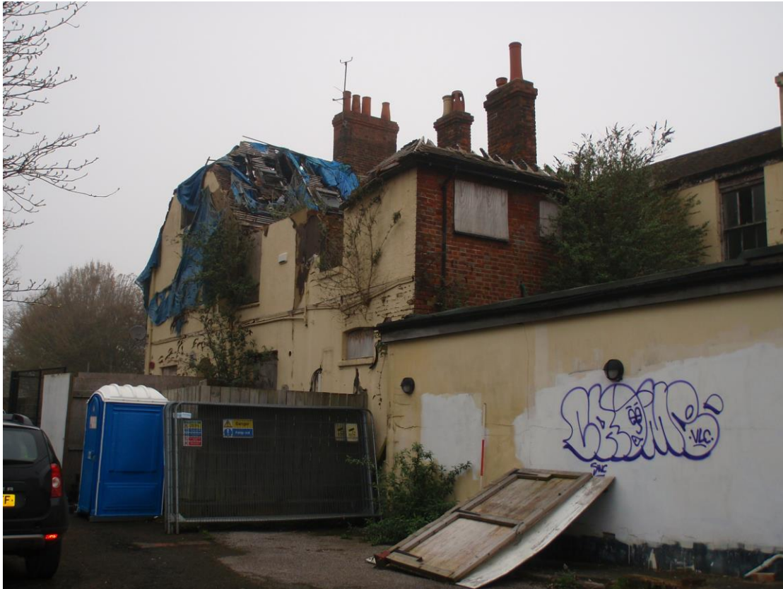
Plate 6. View of rear of Prince Albert (looking north)
